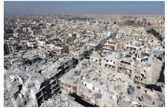
An aerial view of the buildings destroyed by the Assad regime forces and Russian army in the Tariq al-Bab neighborhood.
